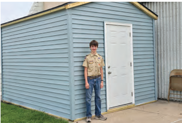
Grand Island Post 53 sponsors Grand Island Troop 119. For his Eagle Scout project, Ethan Millies of Troop 119 planned and constructed a new 10x12 shed for the United Veterans Club.
